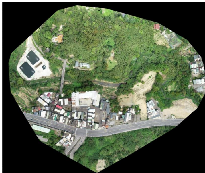
Figure 3.19: DOM After Realignment.
