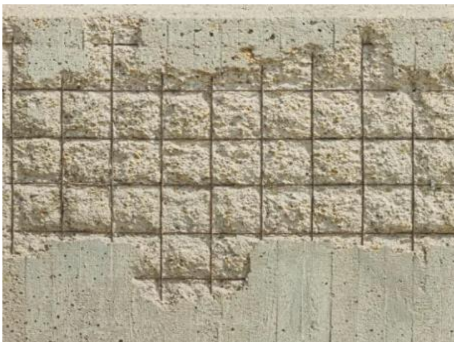
Figure 2.15: Formation of Concrete Spalling (Albrecht, 2019).
