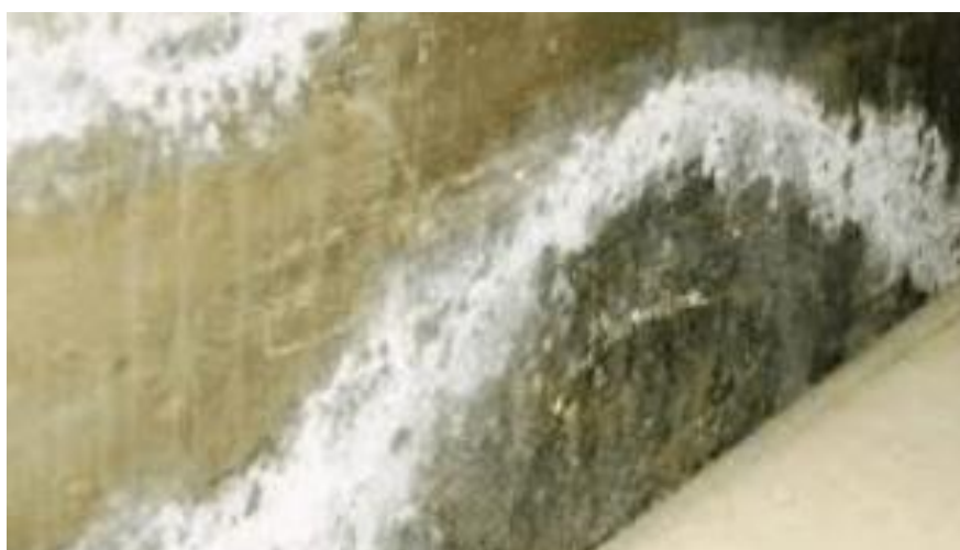
Figure 2.14: Formation of Concrete Efflorescence (Khan, 2020).
