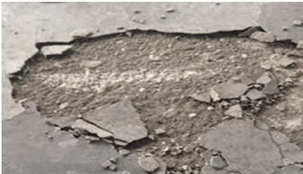
Figure 2.9: Formation of Delamination on Concrete Slab (Khan, 2020).
