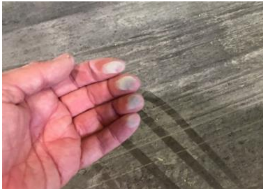
Figure 2.13: Formation of Concrete Dusting/Laitance (Ecoratio, 2019).
