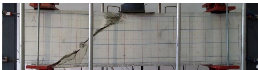
Figure 2.35: Experimental Crack Pattern for Reference Beam (Rai, 2021)
