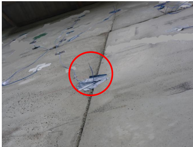
Figure 4.46: Outdoor temperature indicator
