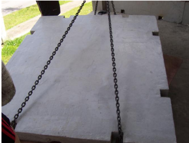
Figure 4.20: Lifting of prototype panel prepared for fixing
