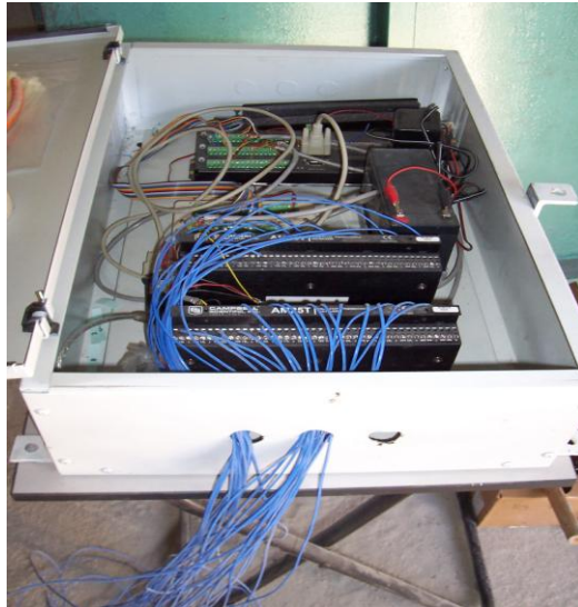
Figure 4.44: Thermocouples connected to multiplexer and datalogger
