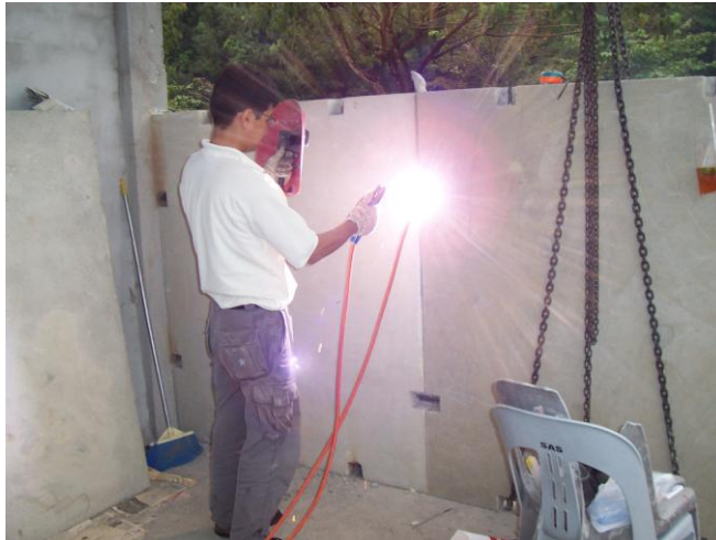
Figure 4.22: Welding work in progress connecting the prototype panels
