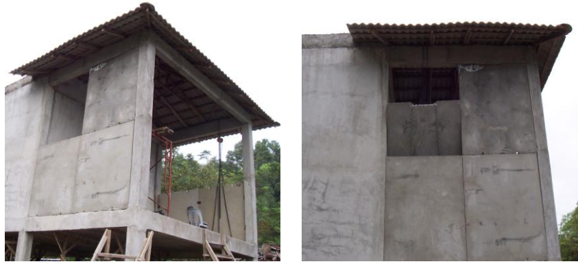
(a) Fixing of sand-based panels
