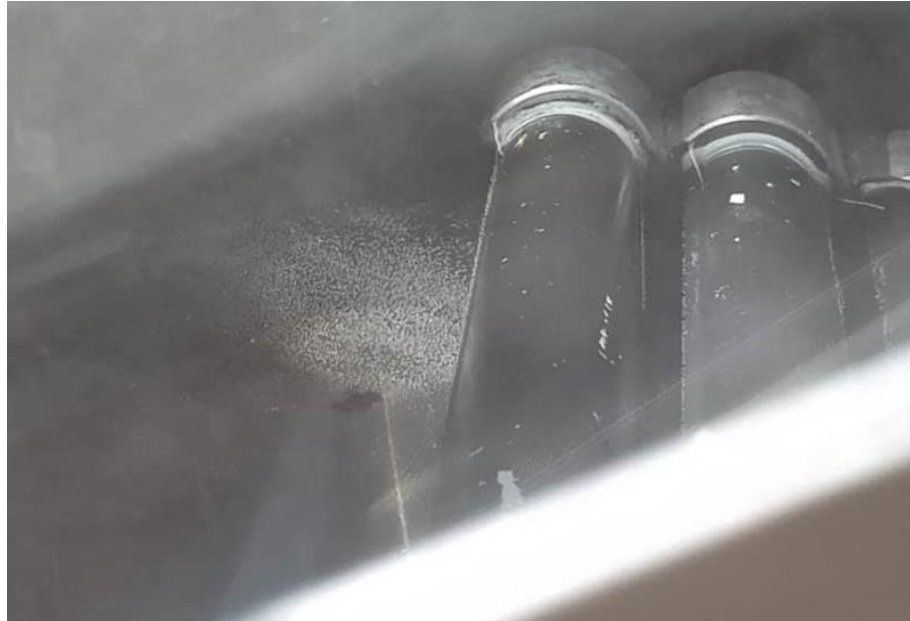
Figure 5.4: Bubbles forming in CSP Solar Still where FRL is used
