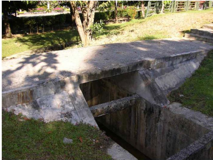
Figure 2.3: Footbridge Constructed with OPS Concrete (Teo, et al., 2006)
