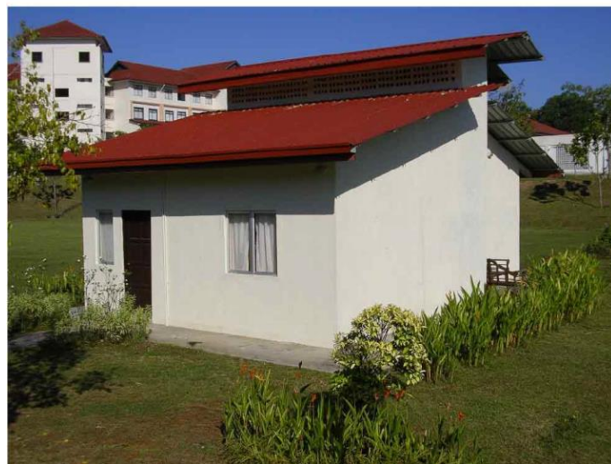
Figure 2.4: Model Low-cost House Built with OPS Concrete (Teo, et al., 2006)
