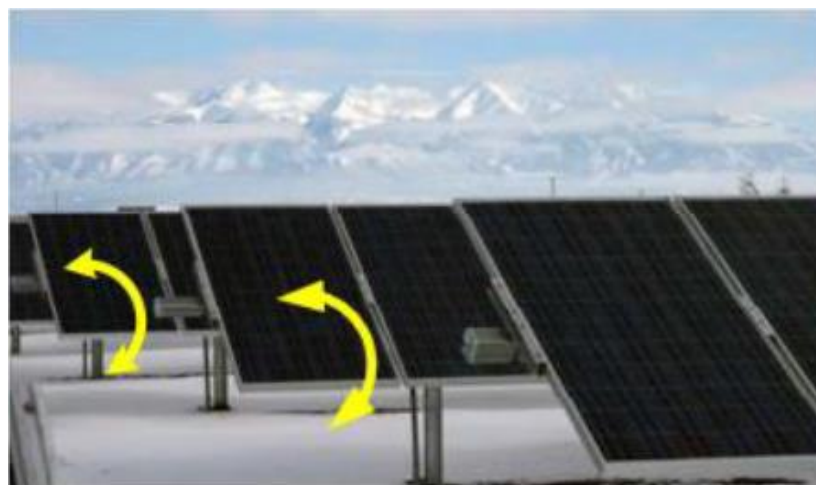
Figure 2.2: Applications of 1 axis sun-tracking (ST) system for solar PV panel (Rockwell Automation, 2011)
