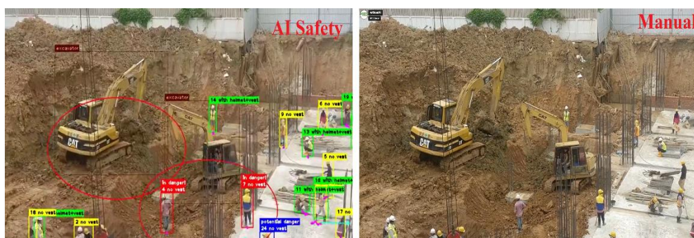
Figure 2.25: AI Safety and manual monitoring on site (mesgroup.asia, 2021).
