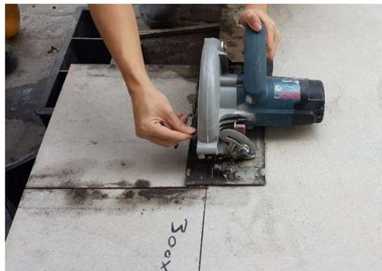
Figure 3.7: Sawing formworks by using a circular saw.
