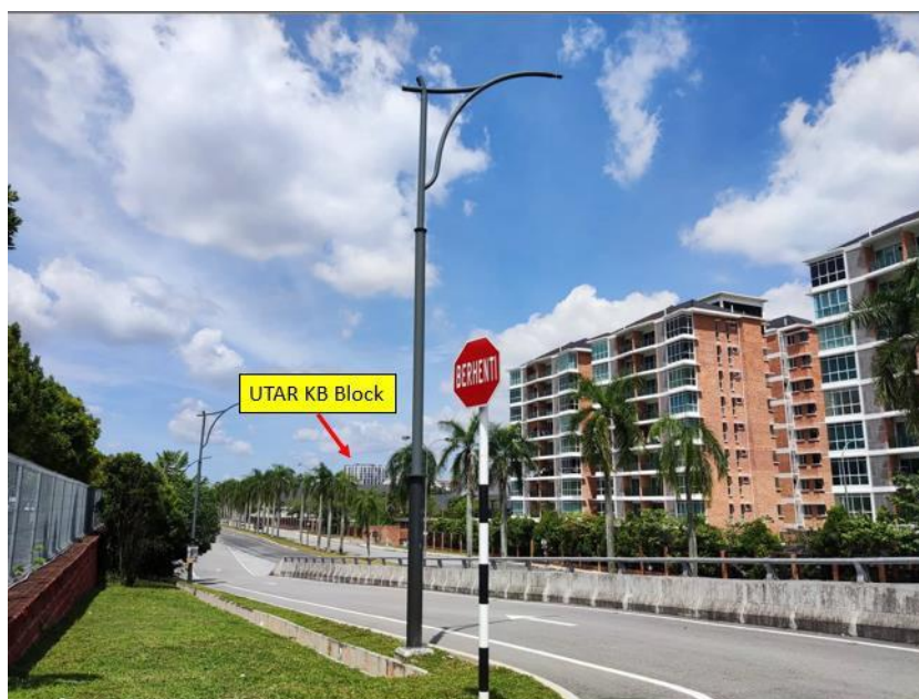
Figure 4.11: Clear Space between Sungai Long Residence with UTAR KB Block.
