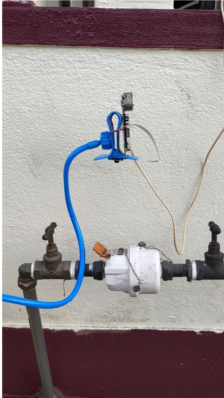
Figure 4.16: Hardware Installation on Water Meter
