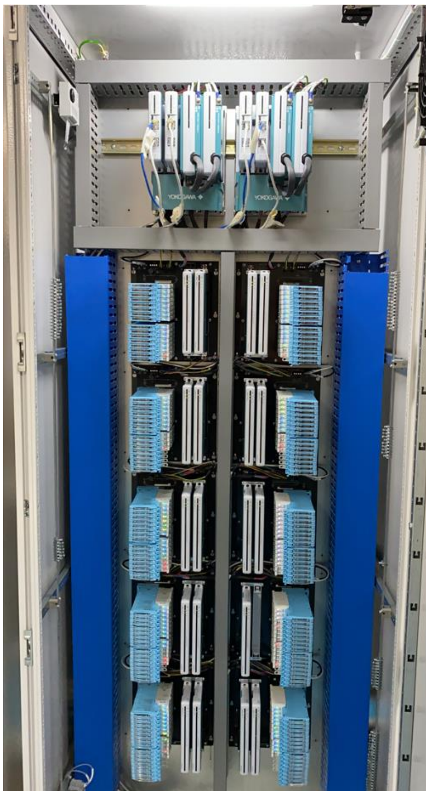
Figure 4.11: Complete configuration Sum5 with Yokogawa DCS
