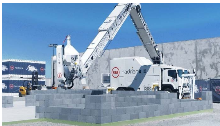
Figure 2.7: Fastbrick Robotics (World Construction Today, 2021)
