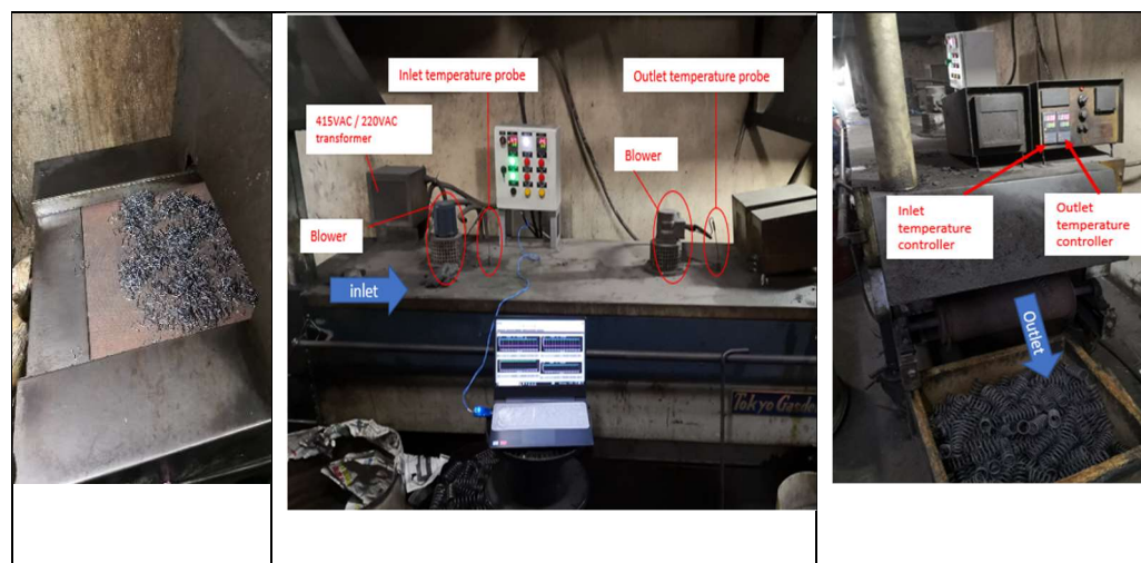
Figure 3.1: Photos of conveyor oven
