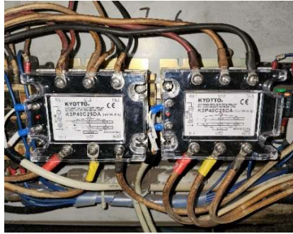
Figure 4.13: Replacement of contactors with solid-state relay
