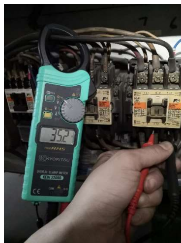
Figure 4.5: Phase-to-phase resistance measurement using clamp meter
