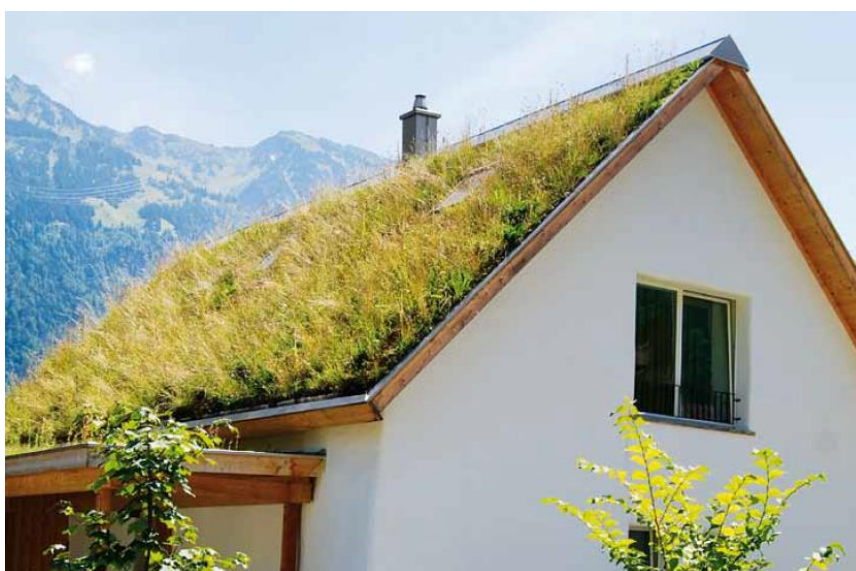
Figure 2.3: Pitched Green Roof (ZinCo, n.d.).
