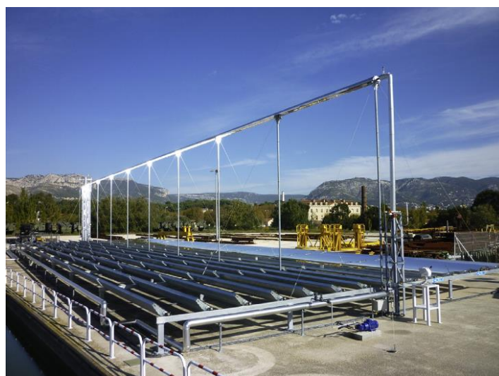
Figure 2.9: The Actual Linear Fresnel Reflector System (Beltagy, et al., 2017 with License Number: 5286060084907).
