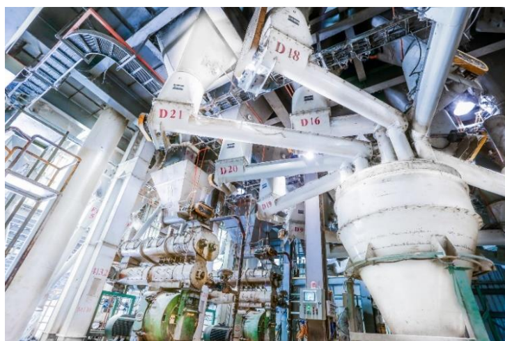
Figure 2.3: Feed Mill in Penang (Kami Farming Sdn Bhd, n.d.).
