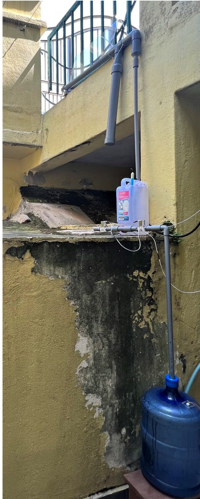
Figure 4.2: Overview of the Design of an Automated RWHS
