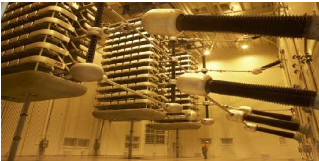
Figure 2.5: HVDC Converter
