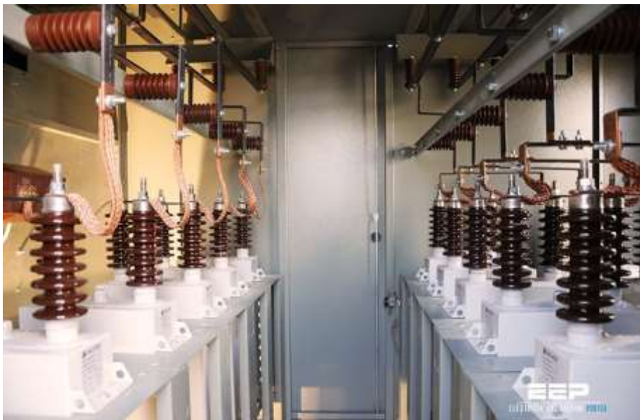
Figure 2.8: Reactive Power Source
