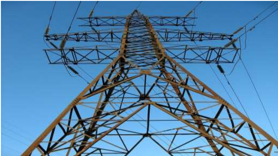
Figure 2.18: Lattice Power Transmission Tower
