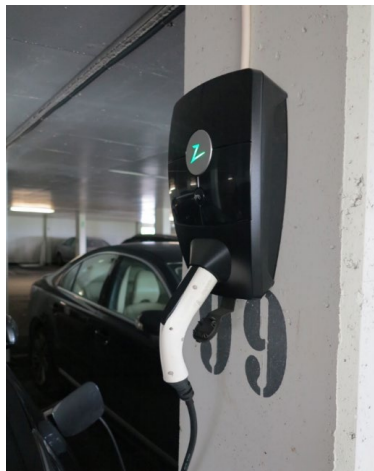
Figure 2.5: Electric vehicle charger installation in car park (Brandt and Glansberg, 2020)
