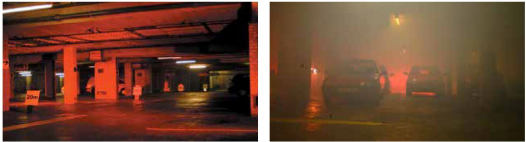
Figure 2.19: Smoke clearance system tests at Bristol car park (Colt International, 2015)
