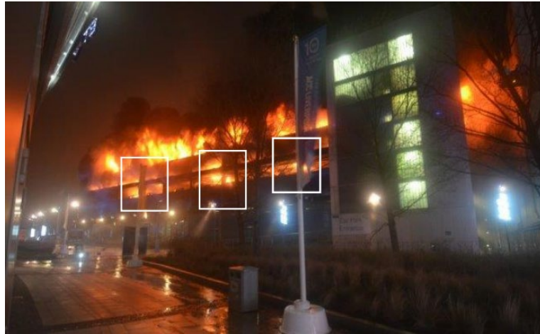
Figure 2.8: King's Dock car park fire (Merseyside Fire and Rescue Service, 2018)
