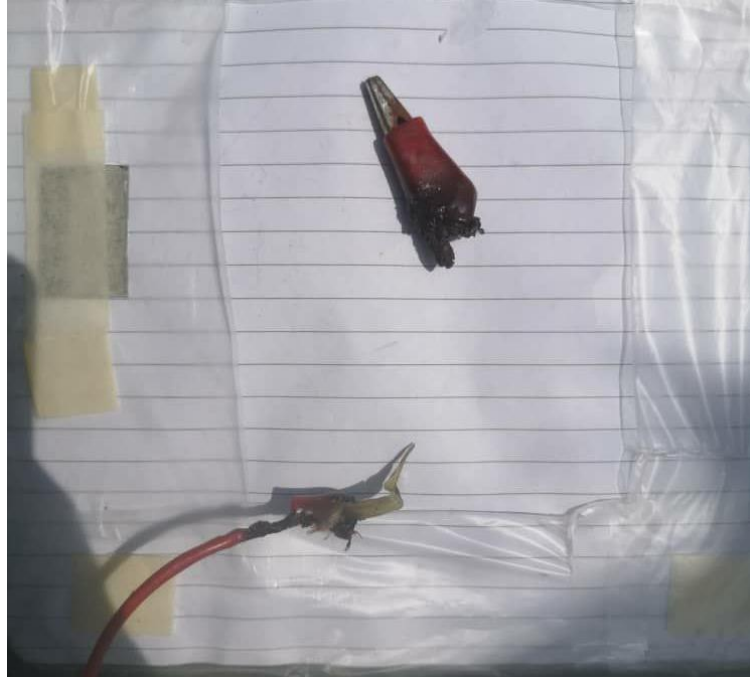
Figure 4.34: Burnt and broken crocodile clip cable from GPV
