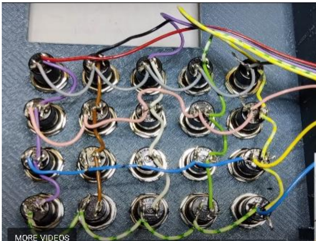
Figure 1.6: The Wiring View of Crumble Deck's Buttons (Arduino Team, 2021).
