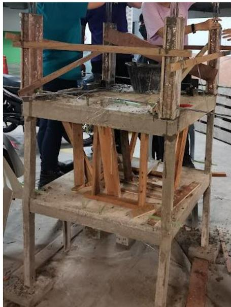
Figure 3.27: Concrete Casting for Third Floor Columns.
