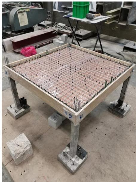
Figure 3.25: Preparation of Concrete Casting for First Floor Beams and Slab.
