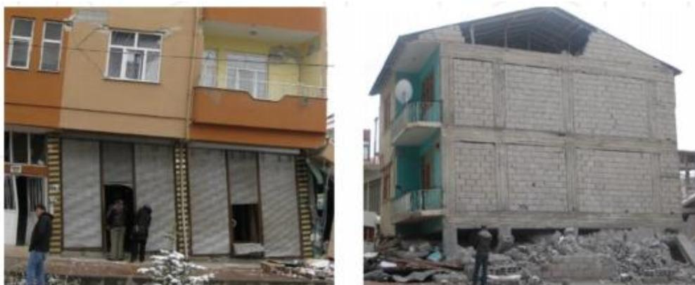
Figure 2.2: Inter-storey Drift due to Weak Storey Mechanism during the Van Earthquake (Yon, et al., 2017).
