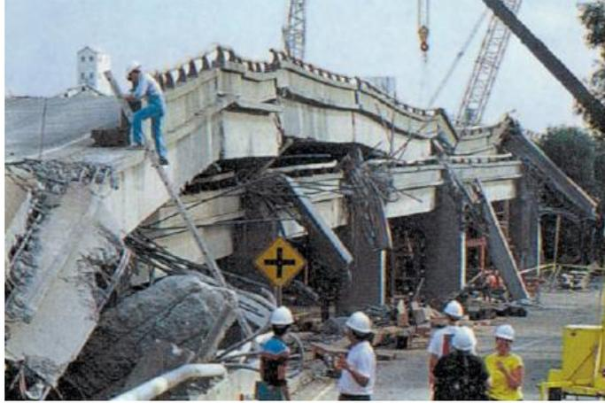
Figure 2.1: Part of the Cypress Freeway in Oakland, California, Collapsed during the 1989 Loma Prieta Earthquake (Earle, 2015).
