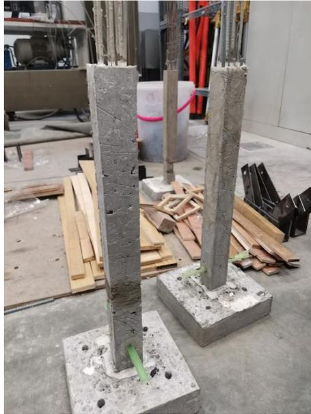
Figure 3.24: First Floor Columns Cast.
