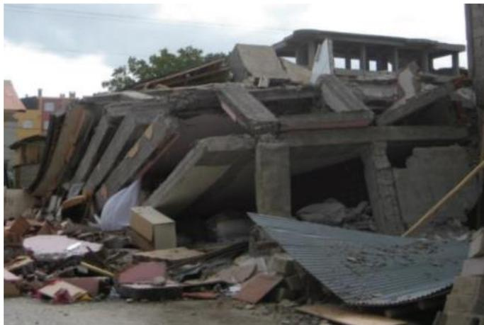
Figure 2.3: Failure Mechanism of Strong Beam-Weak Column during the Van Earthquake (Yon, et al., 2017).
