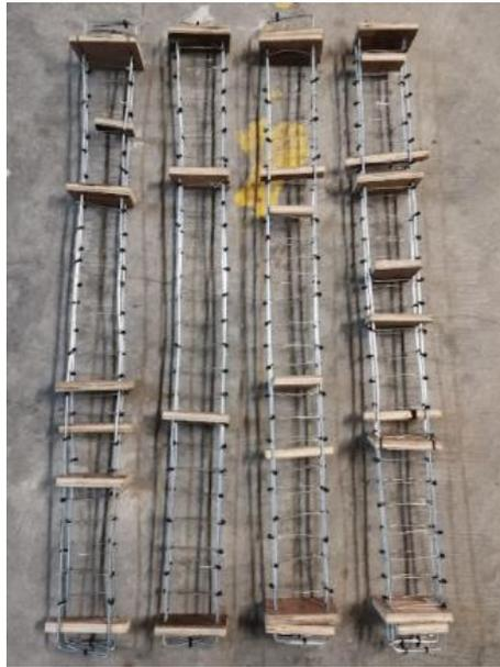
Figure 3.20: Beam Reinforcement.
