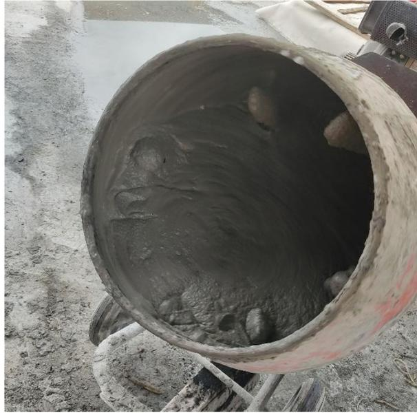
Figure 3.13: Thorough Mix of Foam and Concrete.
