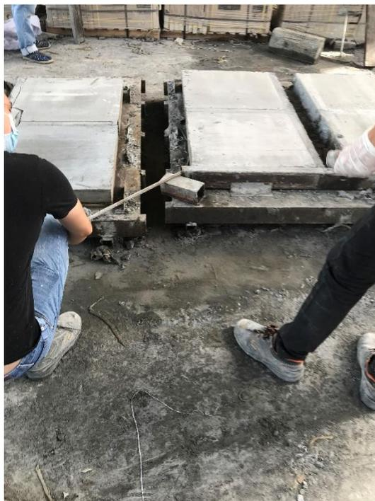
Figure 3.21: Demould of Concrete.
