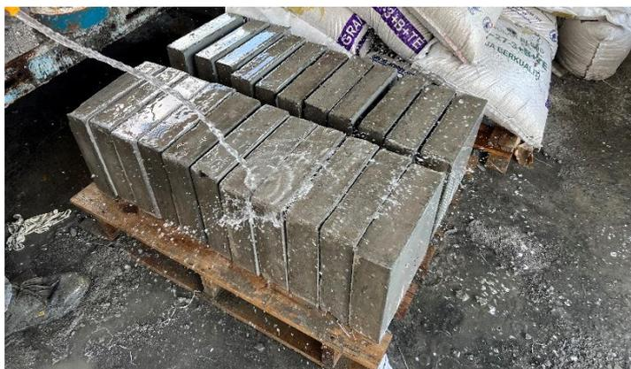
Figure 3.22: Curing of Concrete.
