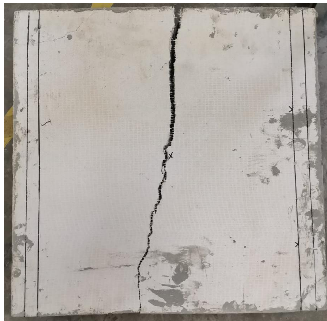
Figure 4.18: Specimen's Condition at Ultimate Failure.
