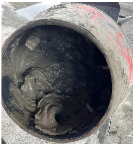
Figure 3.5: Concrete Mixing Process.
