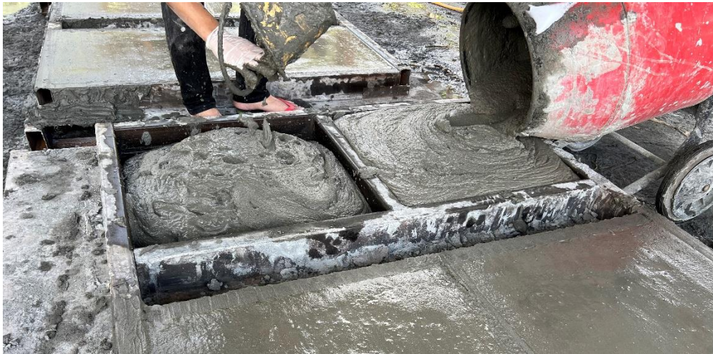
Figure 3.6: Concrete Casting Process.
