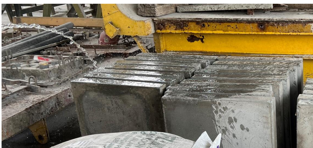
Figure 3.7: Concrete Curing Process.
