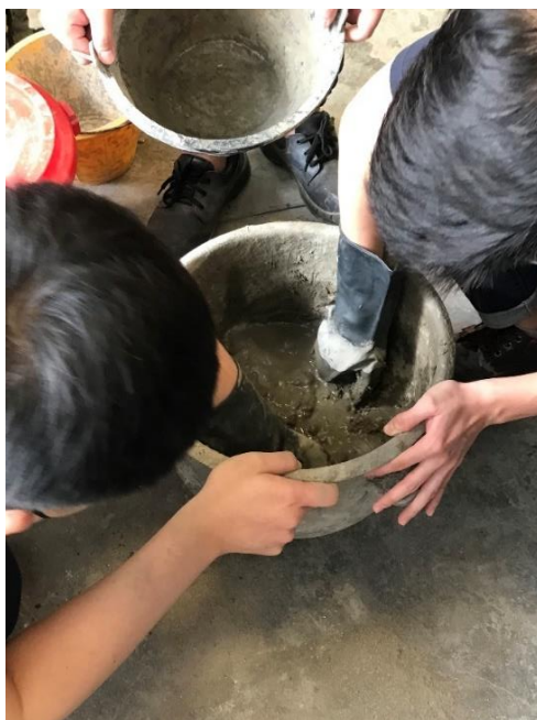
Figure 3.21: Mixing of Dry Mix with Water.
