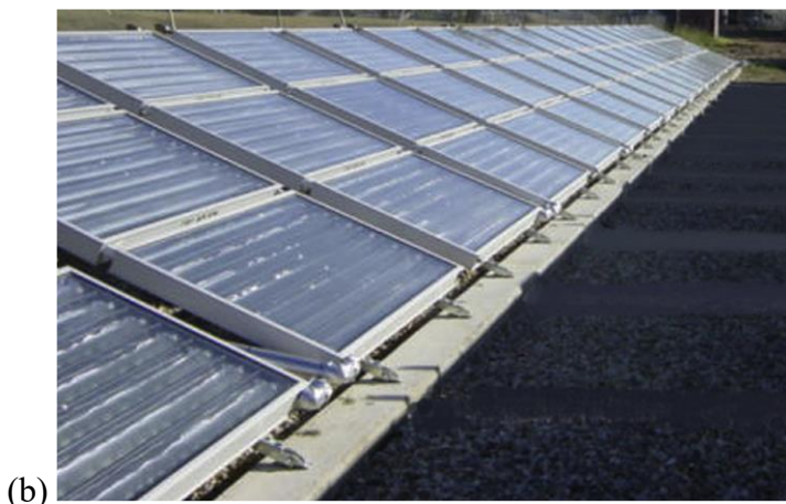
Figure 2.11: CPC panel collector with cylindrical absorbers: - (a) Schematic diagram (b) Photo
