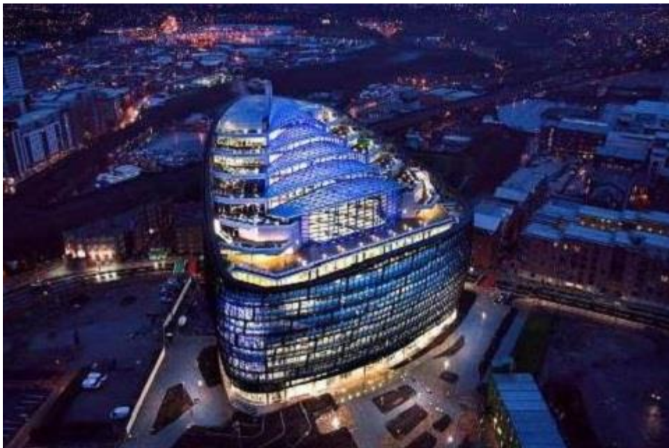
Figure 2.1: One Angel Square, Co-operative Group HQ, Manchester, UK
