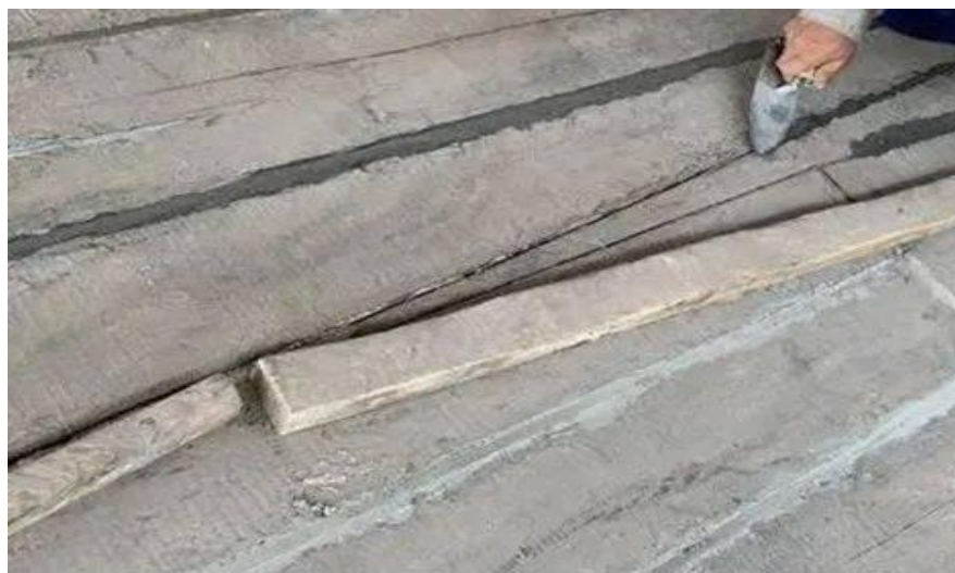
Figure4.4:Plastering at the joints of the roof panels (Source: http://society.sohu.com/a/576510128_121106842 )
