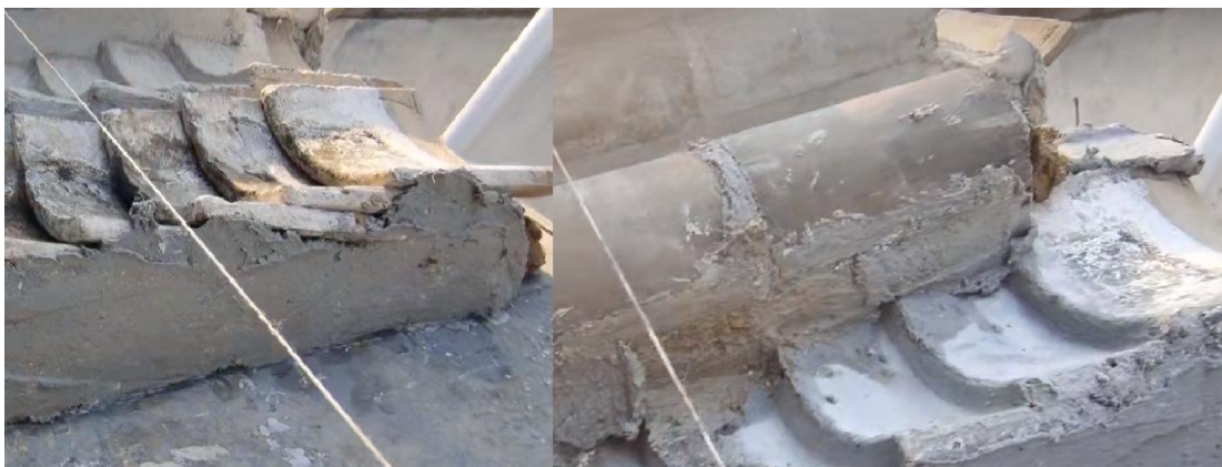
Figure 4.6: Install roofing tiles
