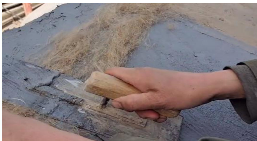
Figure4.5:The fibers are mixed with the slurry, compacted, and dried (Source: https://www.bilibili.com/video/av502740649/?vd_source=d10cec5bb9d10ac220b34f0aca2add2c )
