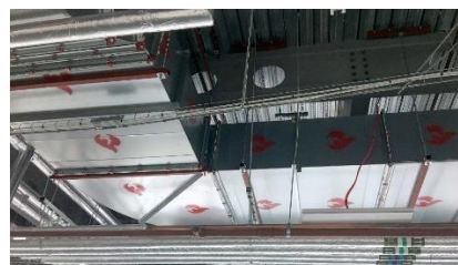
Figure 1.3: Extraction Ductwork (Fire Trace, 2022).
