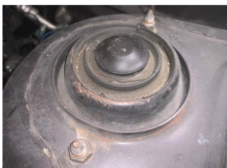
Figure 4.4: Cracks can be Observed on the Mounting Bushing.
