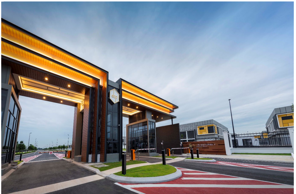
24-hour Security Guard House @ Eco Business Park V
