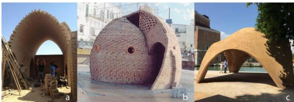
Figure 3: Examples of adobe structures, a) vault, b) dome, c) shell structure (Mintus, n.d.).
