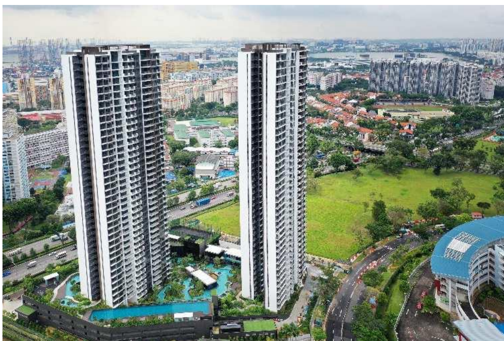
Figure 9: View of the completed project (Seng et al., 2021).
