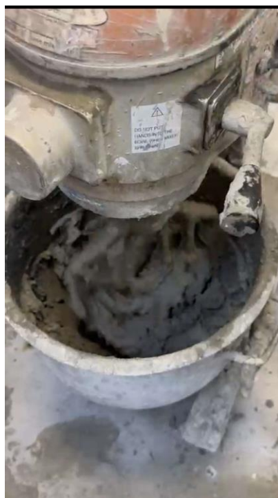
Figure 3.5: Concrete Mixing Process.
