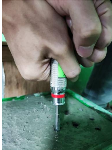
Figure 3.28: Inserting Penetrometer to the Concrete.
