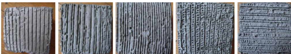
Figure 2.3: Pattern of Roughness Texture on Concrete Surface (He et al., 2017).
