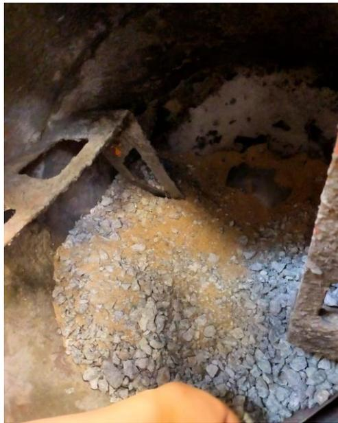
Figure 3.13: Dry Mix in Mixing Machine.
