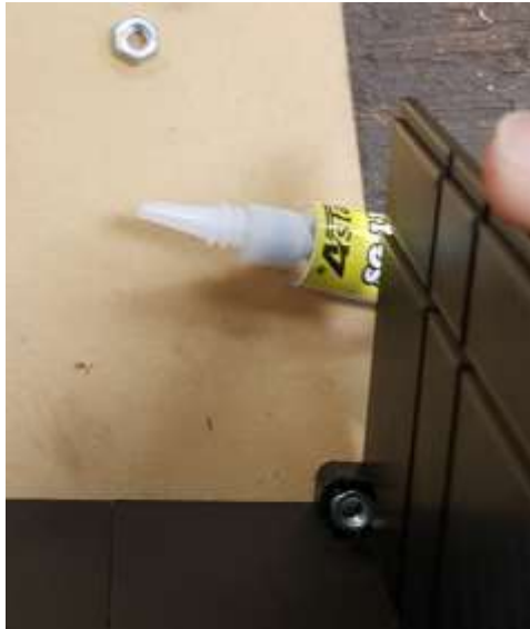
Figure 4.14: The M4 Nuts Are Fixed at The Corners of The Assembled Battery Case Using Strong Adhesive.
