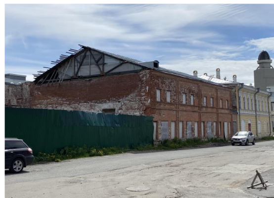
Figure 2.1.7: Main façade of the cinema “Sever” – fixing point II
