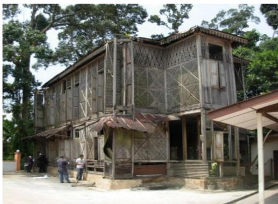
Figure 1.1.2: Ihsaniah Iskandariah Mosque before conservation (2009)
