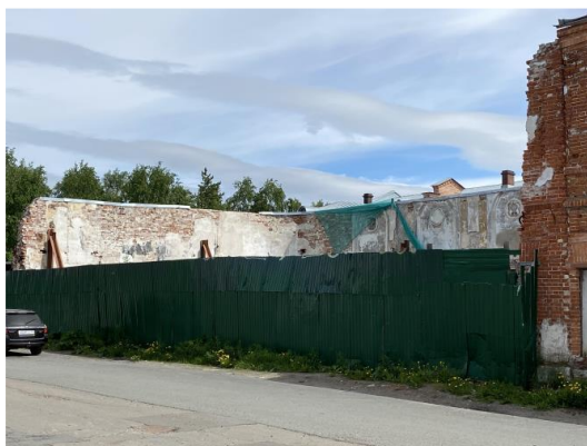
Figure 2.1.6: Main façade of the cinema “Sever” – fixing point I
