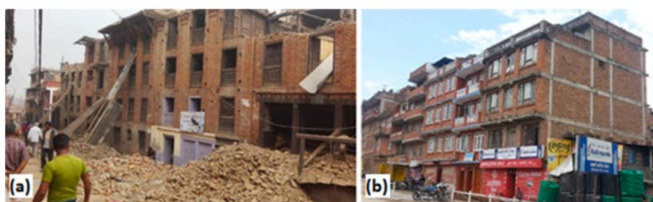
Figure 2. 15: Buildings based on structure type: (a) masonry buildings; (b) RC buildings.
