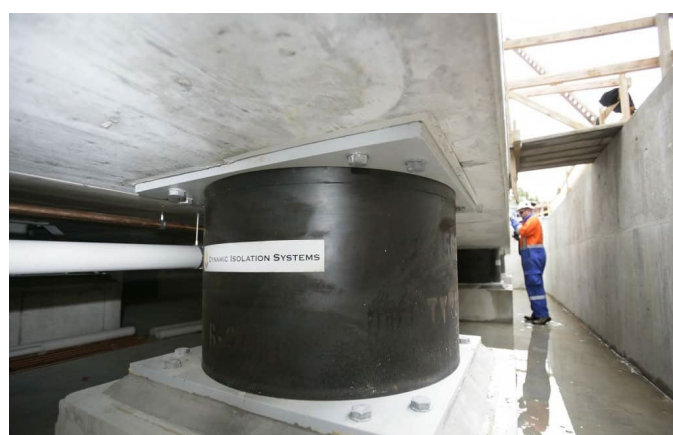
Figure 2. 20: Base isolation for a building (Anand, 2016).
