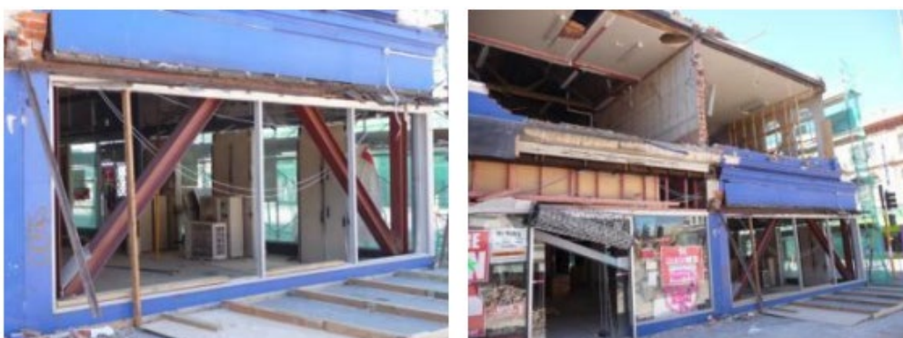
Figure 2. 14: Braced frame as a retrofit to unreinforced masonry building.
