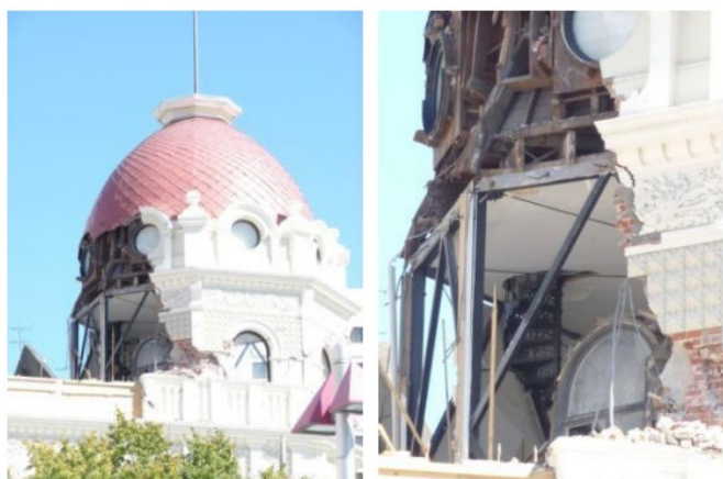
Figure 2. 13: Braced dome at top of Regent on Worchester Building.
