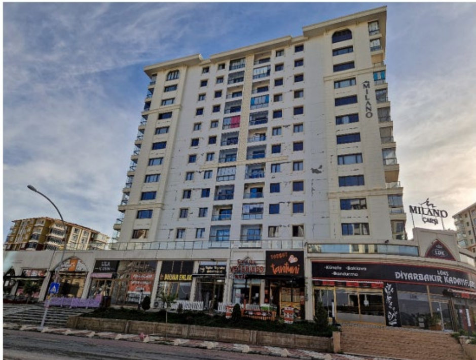
Figure 2. 5: Facade view of the building.
