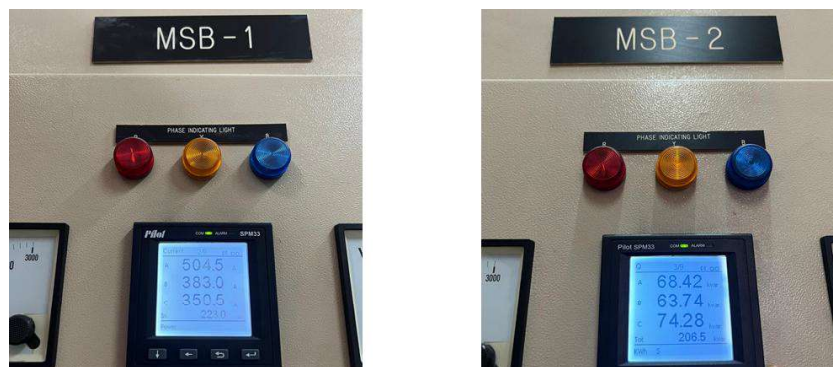
Figure 3.2: SPM33 digital power meters (MSB1 and MSB2) installed at UTAR KA Block for load monitoring.
