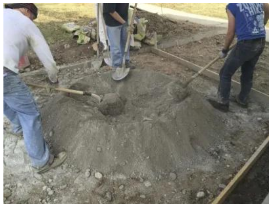
Figure 2.34: Integral Mixing Method (The Constructor, 2018).
