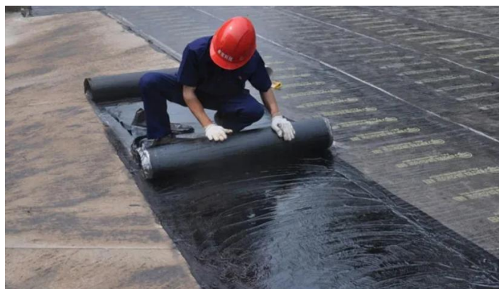
Figure 2.32: Sheet Membrane Method (Constro Facilitator, 2020).
