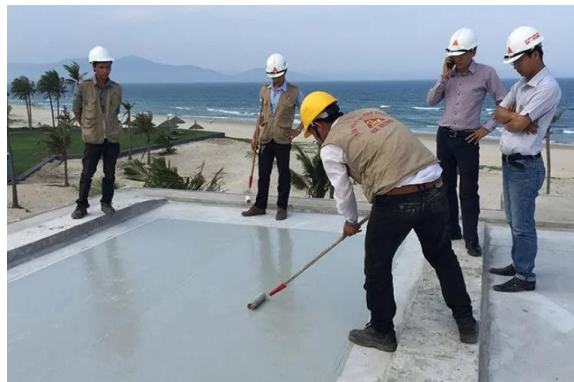
Figure 2.33: Liquid Membrane Method (Constro Facilitator, 2020).
