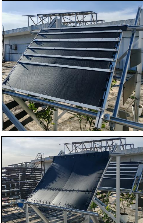
Figure 3. 9: Panel installation on the PV rack
