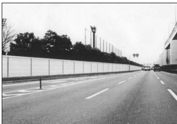
Figure 2.7: View of soundproof highway walls coated with \text{TiO}_2 photocatalysts for the elimination of \text{NO}_x
