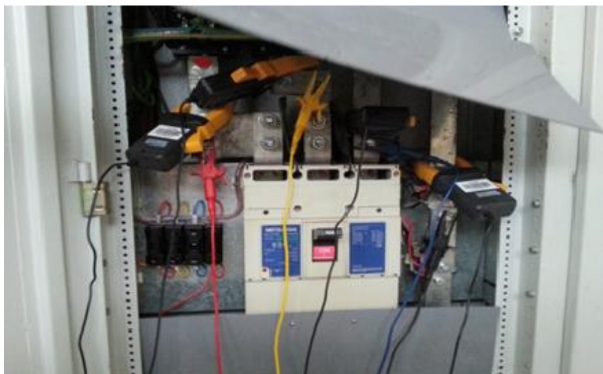
Figure 3.3: Clamping Onto Live Busbars
