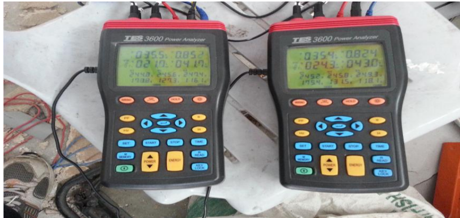
Figure 3.5: Alternative Use of Two Power Analyzer
