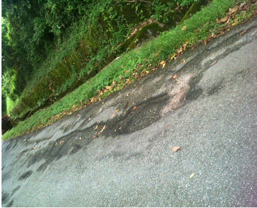
Figure 3.3: Potholes on the road.
